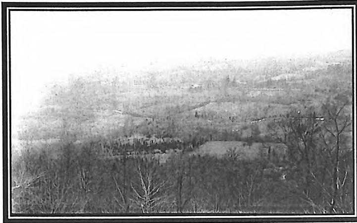
This serene, peaceful valley, full of working farms, orchards and fields was soon to become a cacophony of noise with the removal of trees and homes and the beginning of construction of the "Totoket Dam" as it was known at that time. The little river in the center of the photo is probably "Crooked Brook."
