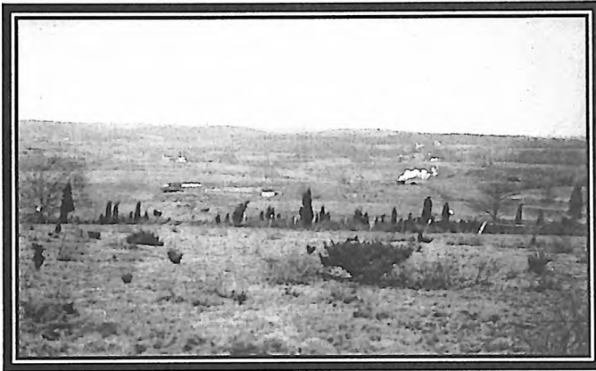
The photo shows the eastern half of the basin prior to the beginning of construction.
