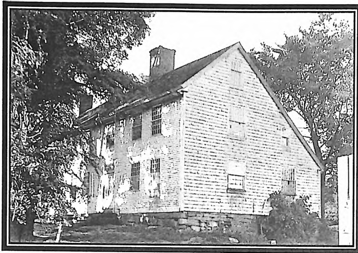
An outside view shortly before demolition. Photo courtesy of the Yale Art Gallery.
