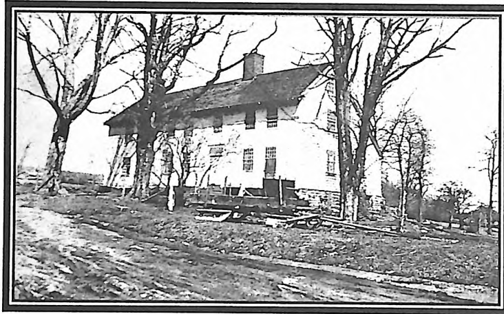
Another view just prior to demolition.
